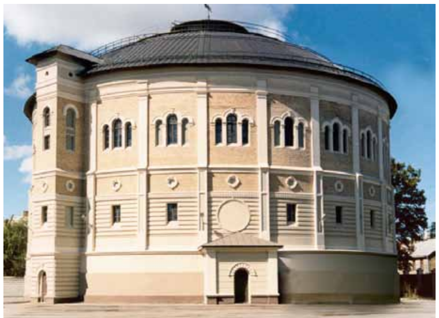
One of the most beautiful and interesting buildings of Riga - the largest and newest gas reservoir that was built for the gas factory in Vagonu Street in 1901.
