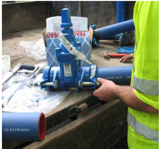
PE pipe with insert is fitted to valve. Note only two bolts required per side for the DN 80, against eight bolts per flange on traditional assembly. No electrofusion required to complete the assembly of the valve
