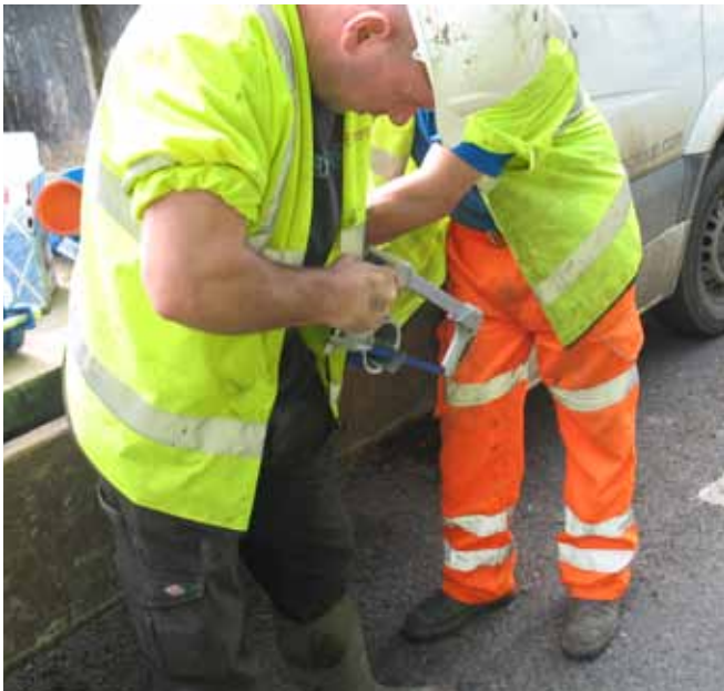
Series 05 stainless steel support bush is inserted and the excessive wedge is cut off
