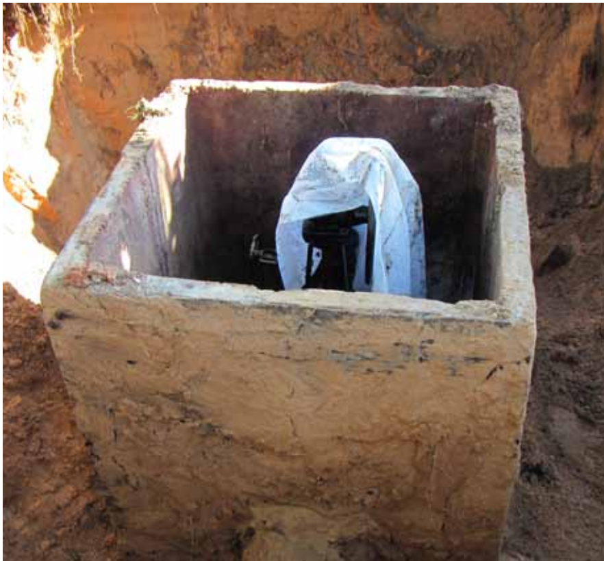
An old valve in a well waiting to be cut out.
