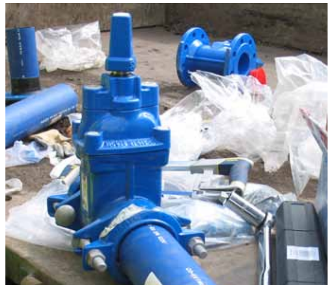
The backing ring is fully torqued to secure the PE pipe. Ready for installation with full end load resistant capabilities.
