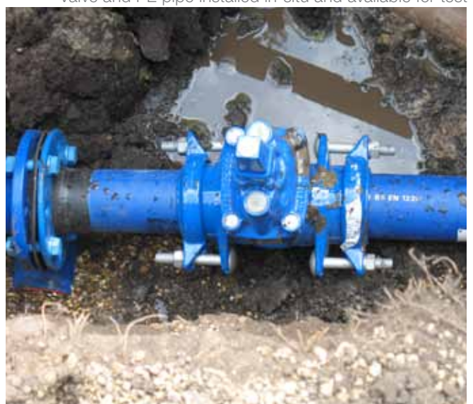
Valve and PE pipe installed in-situ and available for test
