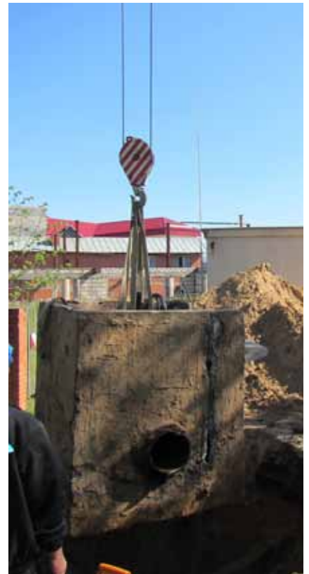
Lifting up the concrete well including the old valve.
