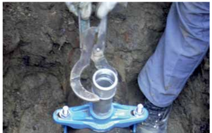
Access to the connection under the airvalve
