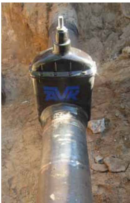
New valve installed and ready to be buried underground.
