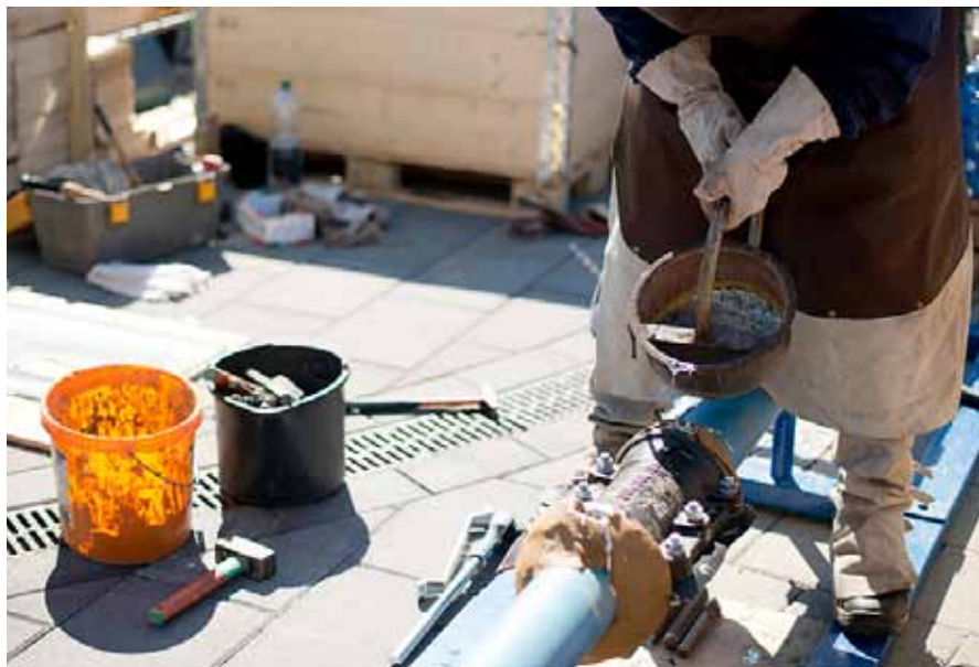
A special discipline - the technique of joining cast iron pipes using cord and molten lead.
