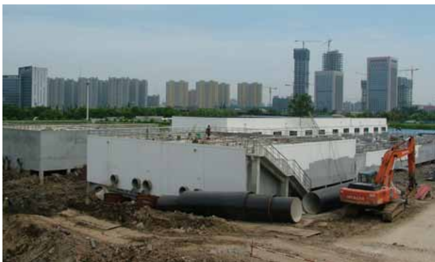
New activated carbon filters.
