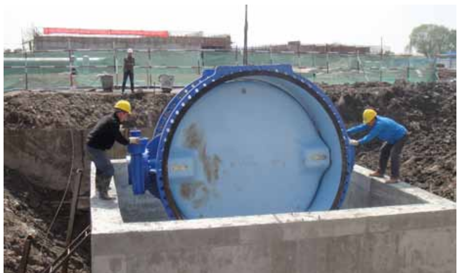
Installing series 756 DN 2800.
