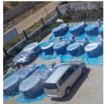
AVK valves on site at HUDA, Division 3.
