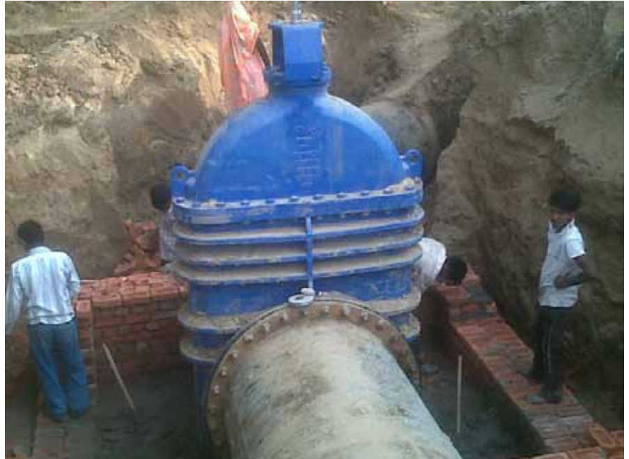
Installation of a DN 1600 metal seated gate valve on site.
