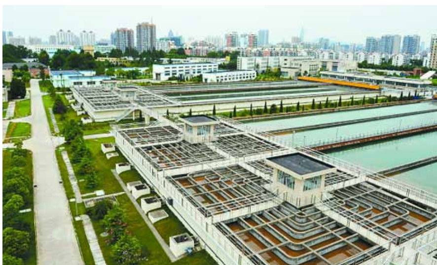
BEIHEKOU Water Treatment Plant operated since 1929.
