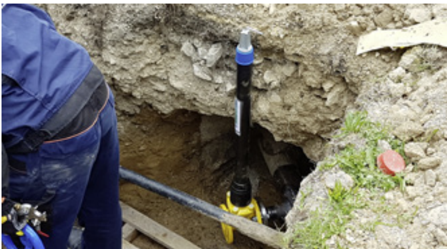
Photo 2 Ready to connect pipe to the end user
