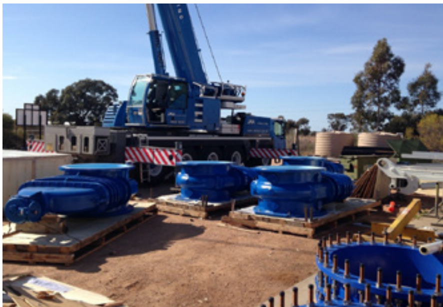
Valves arrive on site in Renmark on 19 August 2015 ahead of schedule
