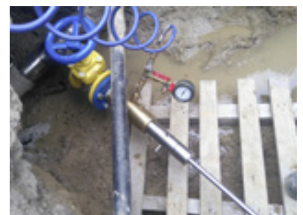
Photo 3 Testing for leakage
