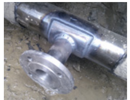
Photo 1 Tee welded on 100 mm steel pipeline
