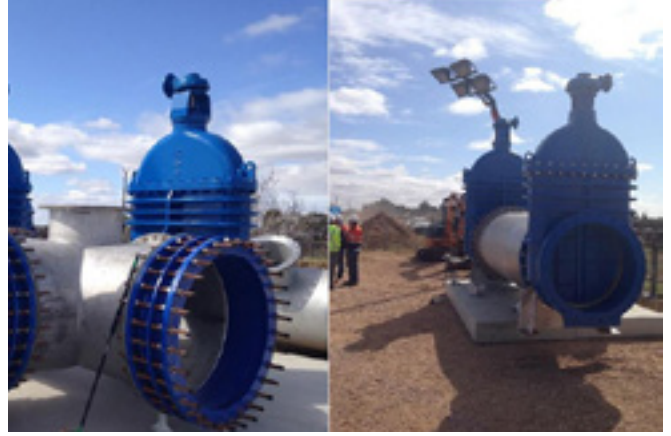
Site 2, Scott Stone (AVK) with some final checks of the valves (4x DN1200 & 1x DN1000) - 26 August 2015.
