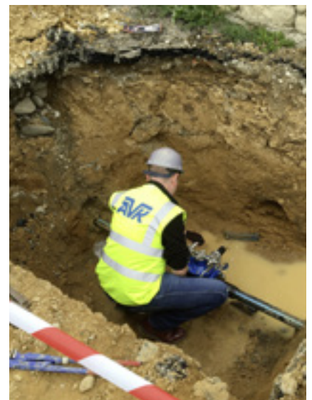
AVK commissioning support in Tbilisi
